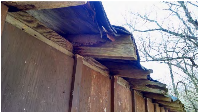
Stan Murray Shelter Roof Condition
