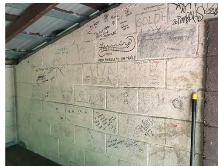
Abingdon Gap Shelter: Before and After
