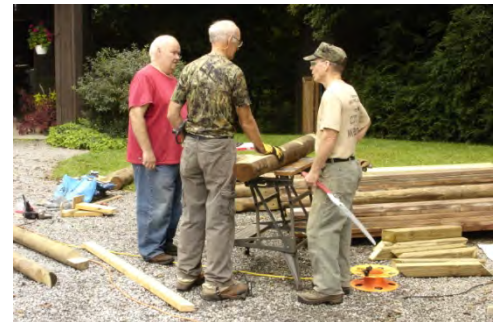
Much sawing and drilling at Carl's house
