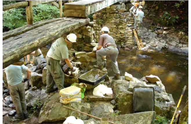
Enlarging rock piers
