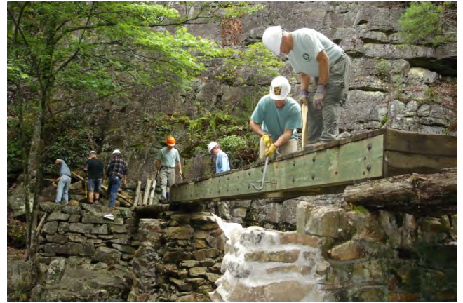
Dismantling the old bridge
