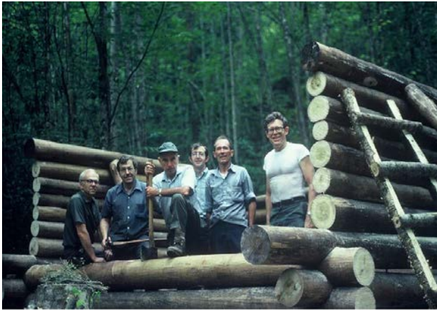
Darrol (second from left) along with other TEHCC members during construction of the Don Nelan Shelter in 1981
