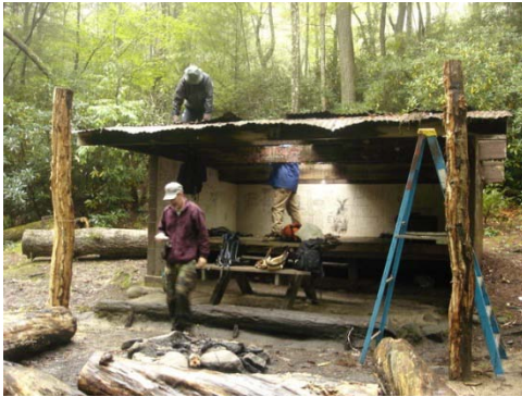
Removing the roof from the old shelter
