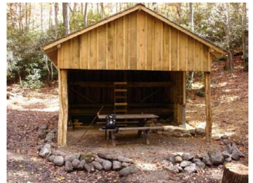
Newly remodeled Curley Maple Gap Shelter
