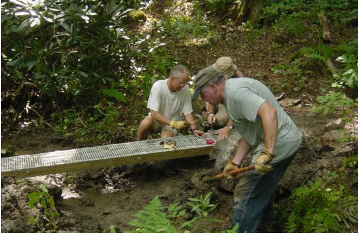
Murdoch, Daryel Anderson and Ted Mowery installing bog bridge, photo courtesy of Ken Buchanan
