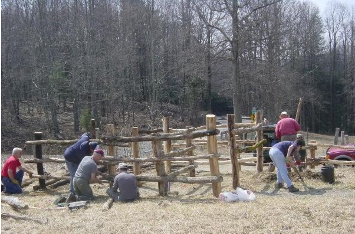
Installing the stile at the Osborne Tract
