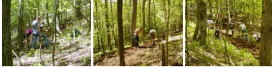
The finished bog bridge, More sidehill construction on Monday
