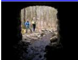
Exiting tunnel under Cades Cove Road
