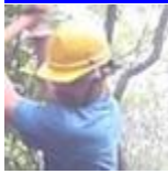
Breaking rock , July 13, 2003 (160KB). Photo courtesy of Steve Wilson.
