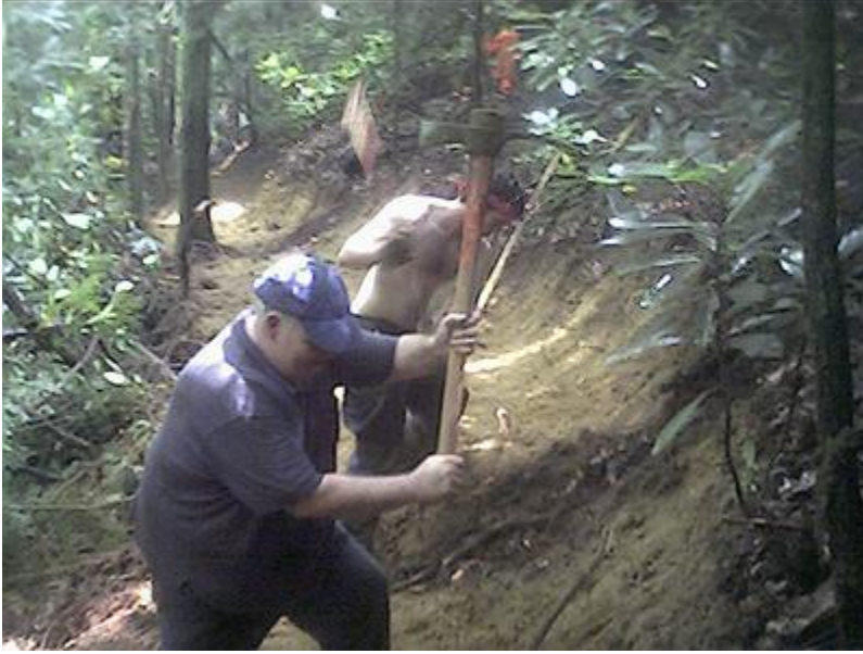
Volunteers constructing new trail on the Elk River Appalachian Trail Relocation
